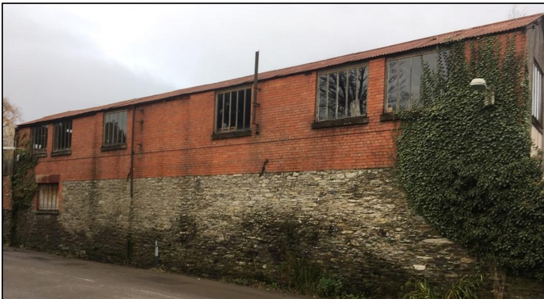
The workshop for horse drawn carriages opened in 1904-5. In its heyday it included a forge for the metal components of the carriages; the open ground floor was used to assemble the vehicles and the upper floor contained the upholstery department. The cast iron pillars that support the gable end of the building are believed to have come from Coalbrookdale, where the Industrial Revolution began.
